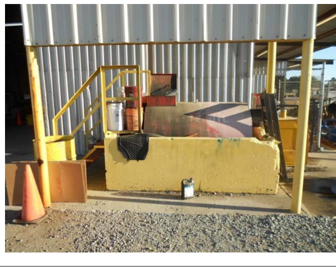
Used oil AST area on the outside of the shop building.
