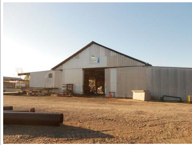
Shop building, facing south.
