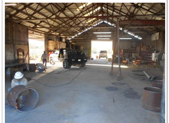
Interior of shop building.
