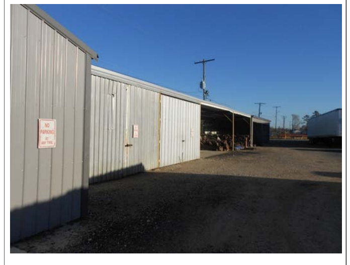
Storage building located along the western boundary of the subject property.
