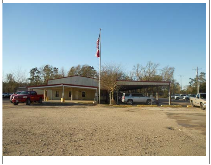
Office building and covered parking located on the southwestern portion of the subject property, facing south.
