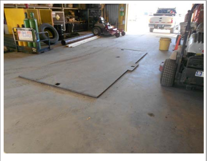
Service pit located in the shop building.
