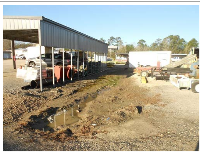
Earthen ditch that traverses the central portion of the subject property.
