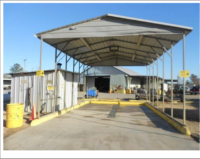
One of two vehicle wash areas.
