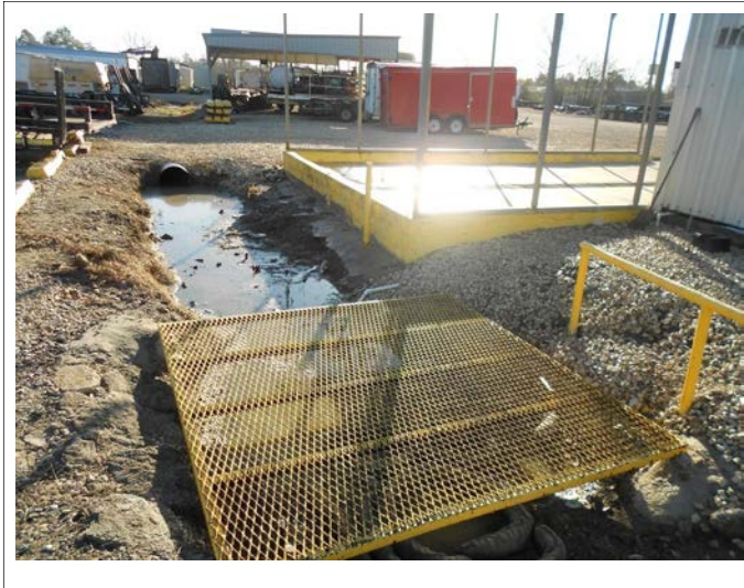
Earthen ditch in the central portion of the subject property near the western vehicle wash area.
