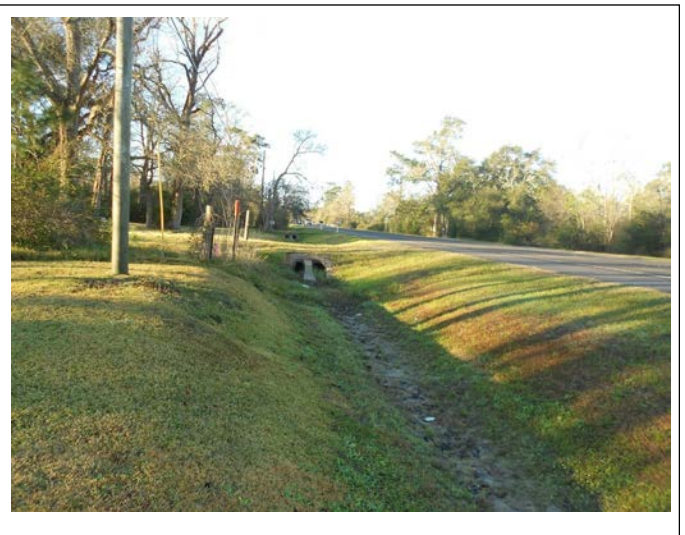
Roadside ditch and Texas Highway 124 frontage, facing southwest.
