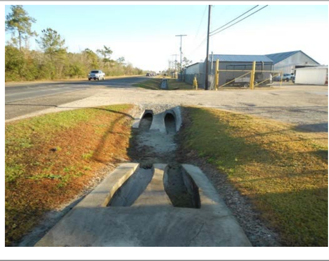
Roadside ditch and Texas Highway 124 frontage, facing northeast.
